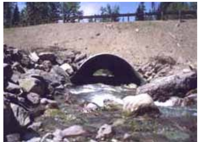
This culvert was reconstructed to allow fish passage.
